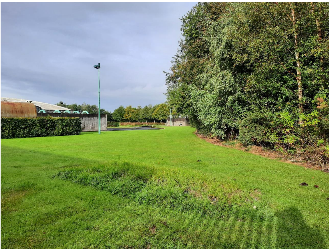
FIGURE 11-10: CORCANREE PS EXISTING EAST END- LOCATION OF PROPOSED STORM TANK PIPE WORK, FACING NORTHWEST
